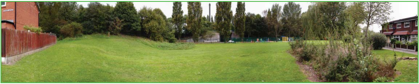
View from Public Open Space East of Shackleton Street showing Gasification stack
